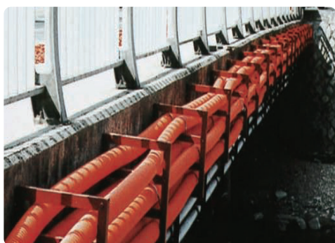
Sub-Duct Coupling after Connection
