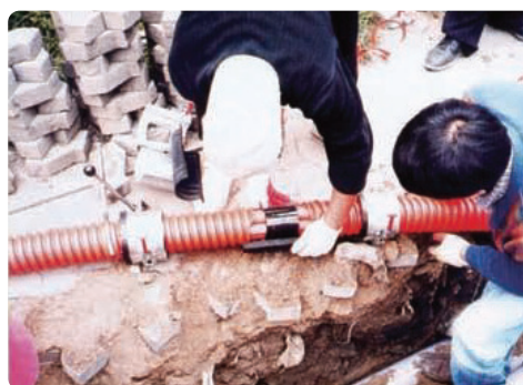
Sub-Duct Coupling after Connection
